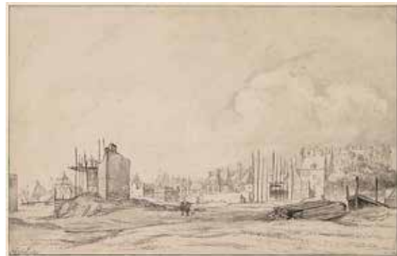
Fig. 18 Jan van Kessel (1641–1680), Demolition of the Heiligewegspoort , 1664, black chalk and gray wash, 19.6 x 30.4 cm. Stadsarchief, Amsterdam, inv. no. 010097006275 (artwork in the public domain)
