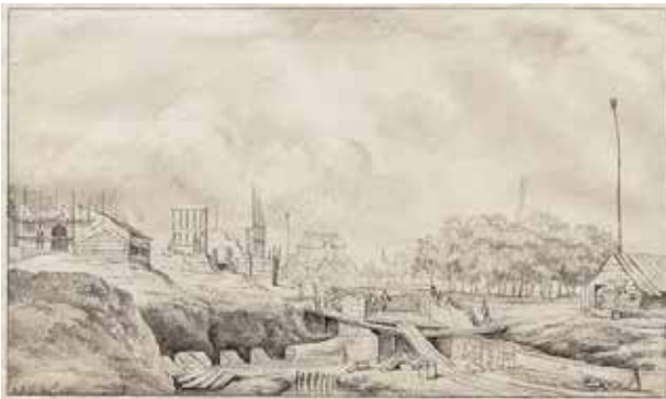
Fig. 17 Jan van Kessel (1641–1680), Demolition of the Heiligewegspoort , 1664, black chalk, pen and gray ink, gray wash, 17.9 x 30.5 cm. Stadsarchief, Amsterdam, inv. no. 010097001725 (artwork in the public domain)
