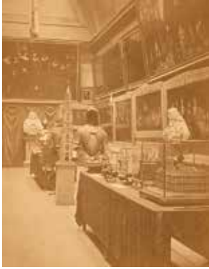
Fig. 27 Pieter Oosterhuis, The Amsterdam Museum of the K.O.G. , 1877, photograph. Amsterdam City Archives, Amsterdam, B00000032800 (Artwork in the public domain; photograph provided by Amsterdam City Archives).
